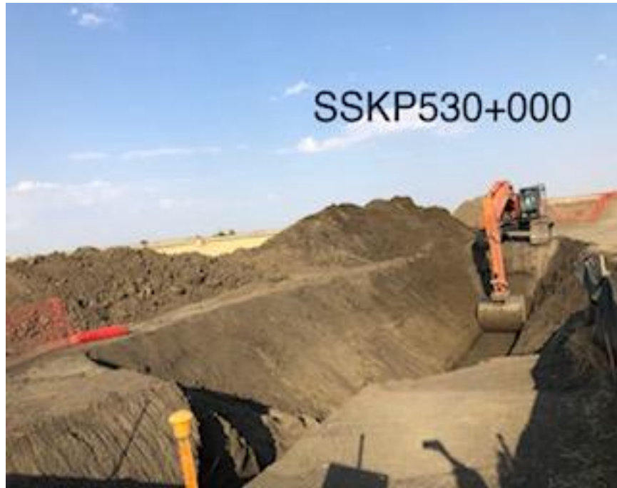
Bell hole excavation at kick off 4m deep near hotlines
