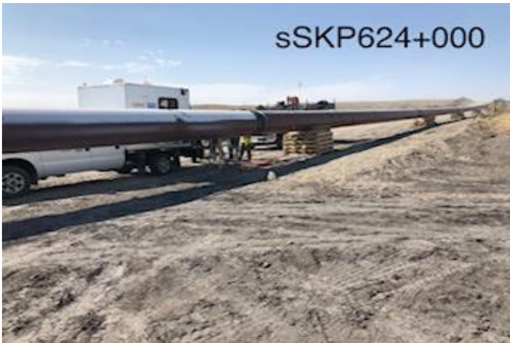
Welding crews complete drag section at Chapleau Lake
