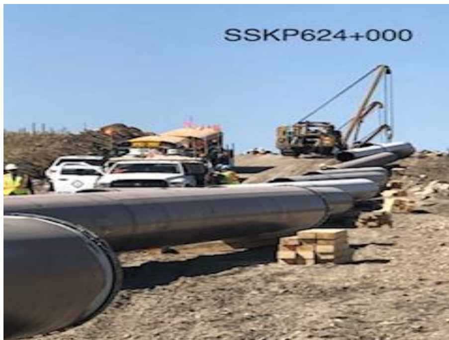
Welding crews at Chapleau Lake HDD drag section
