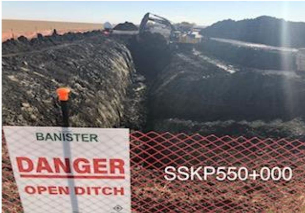
Excavation on SF10
