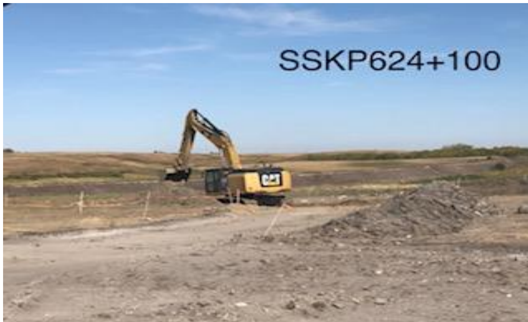
Chapleau Lake Dugout backfill
