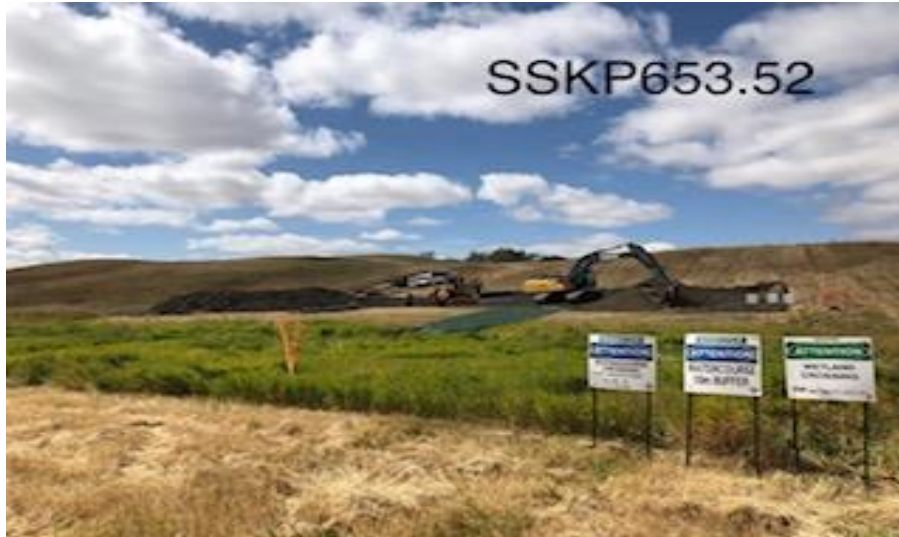
Vipond Creek Top soil stripping and soil separation
